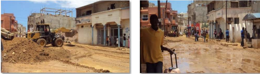
Fig. 6. Filling work of the road no. 241
