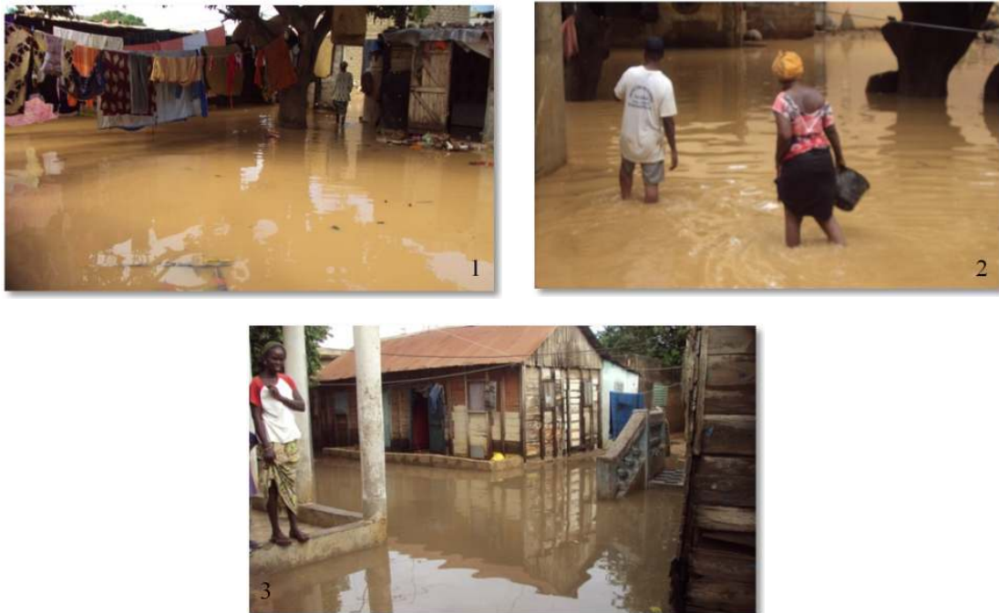
Fig. 7. Houses flooded to the plane (1) city, Touba Ouakam (2) and in the traditional neighborhood Bulgakov (3)
