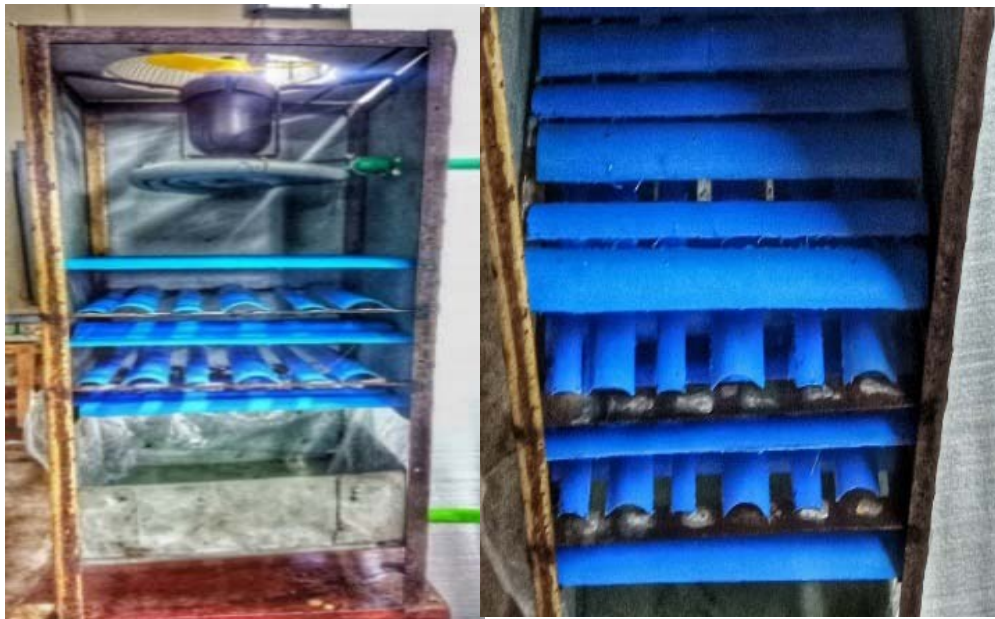
Fig. 7. Cooling tower with inverted u-shaped splash fills
